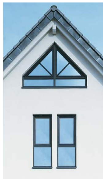
Horizontal muntin bars emphasize the window divisions and optically widen the building
